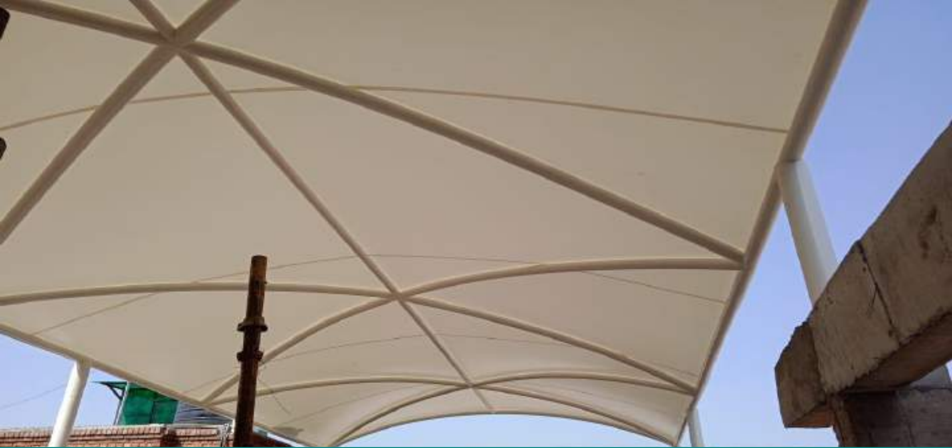
Upgradation of corridor tensile work, Block II, Floor III - Completed
