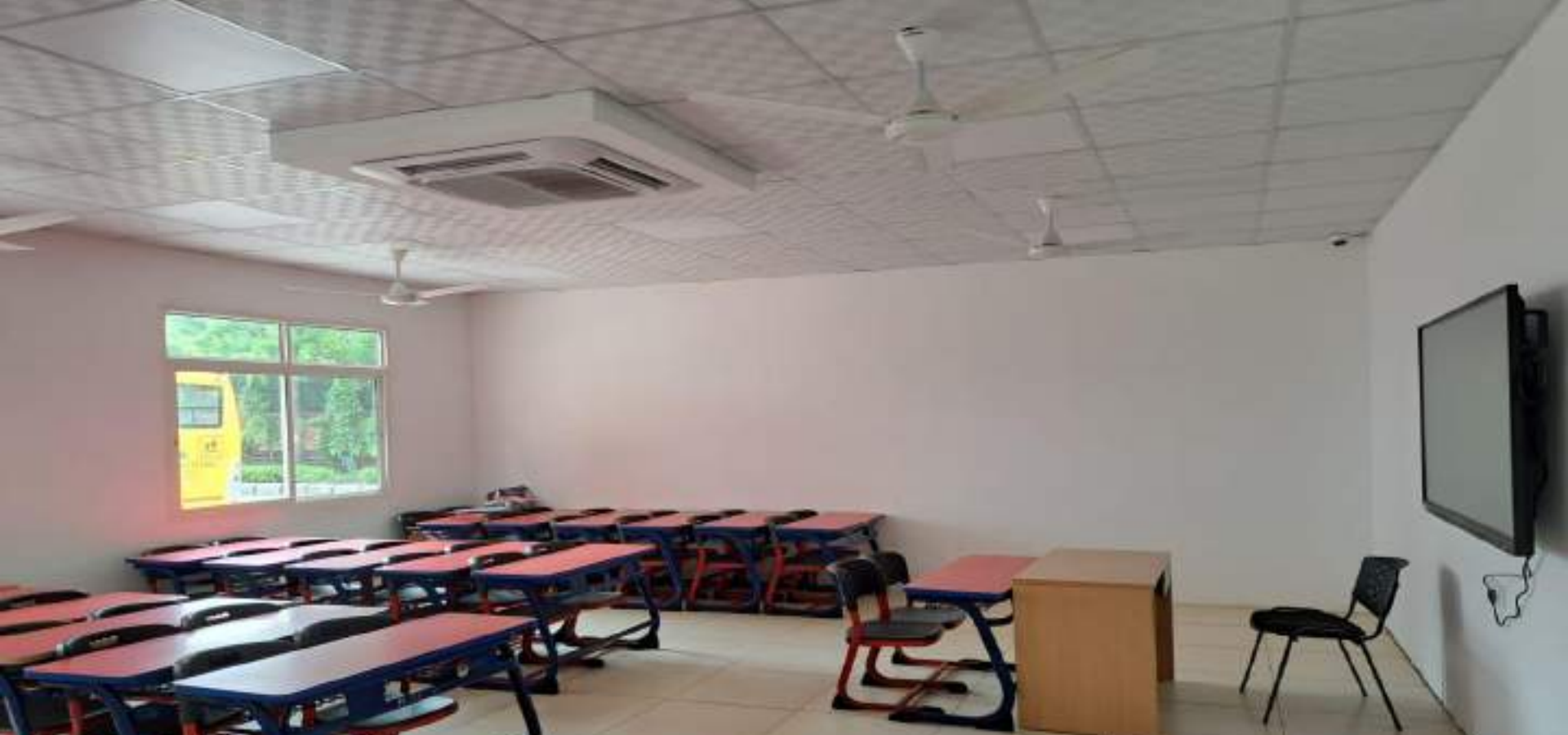
Creation of four classrooms, Ground Floor near gate no 1 - Completed
