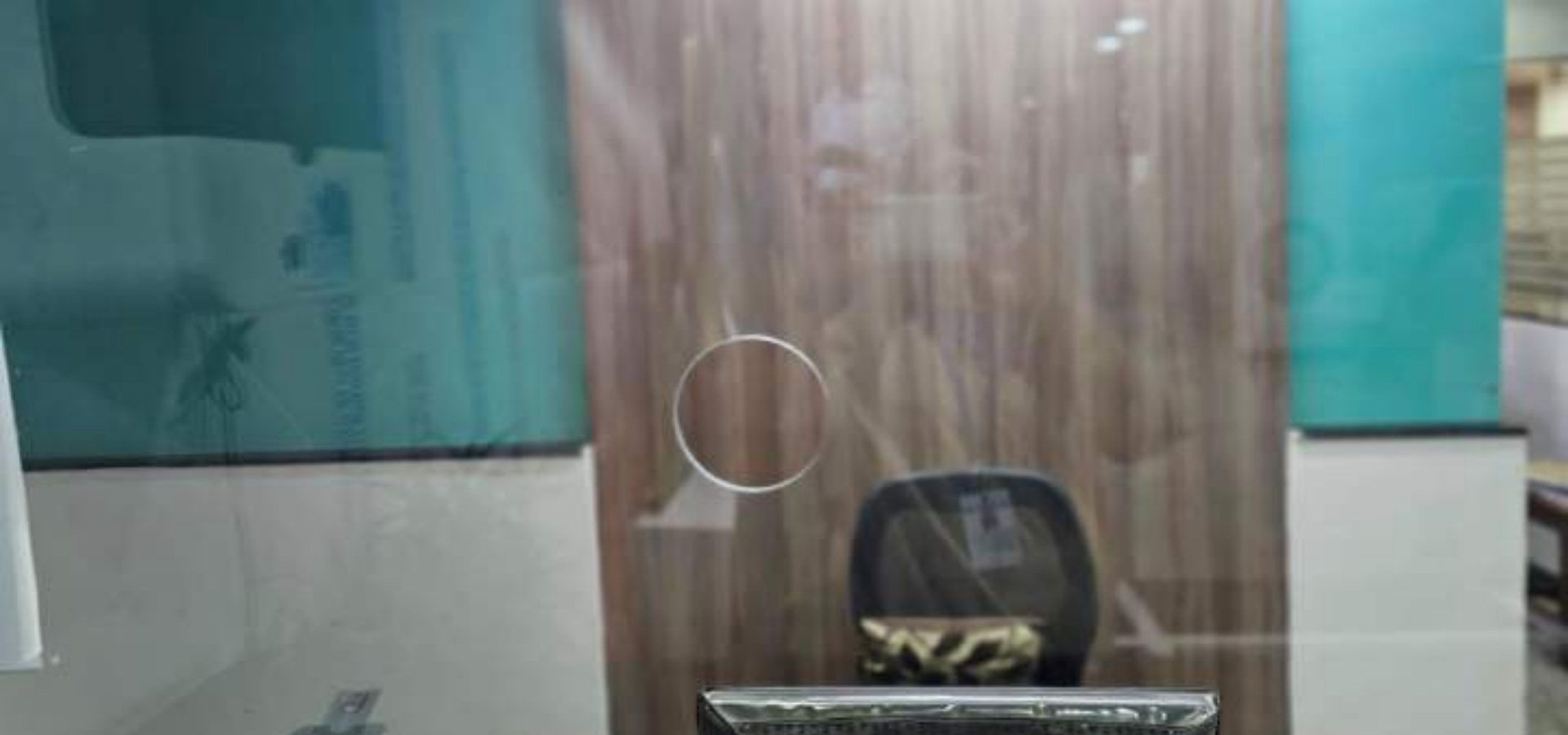
Upgradation of admin office, Ground floor Block II - In progress
