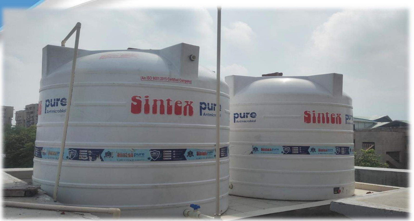
Restoration of damaged roof slab & fitting of tanks-boys' toilet, Block 1
