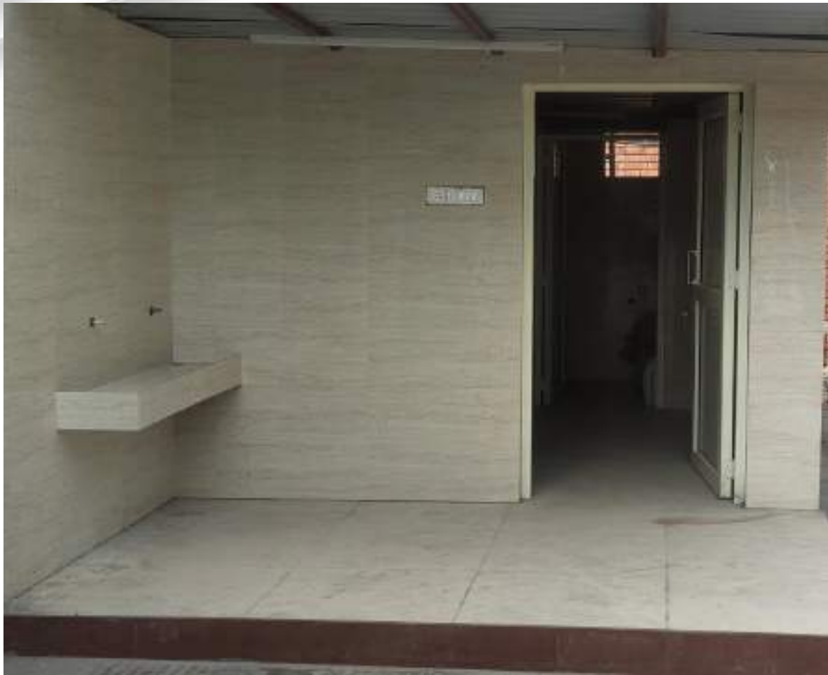
Upgradation of girls toilet at Temporary Block at sector 14 Rohini.
