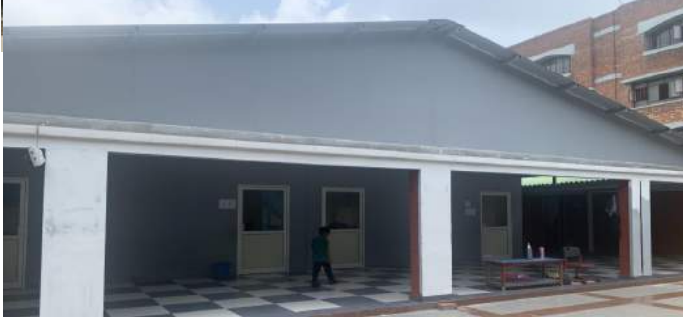
Porta Cabins in Temporary Block at sector 14 Rohini.
