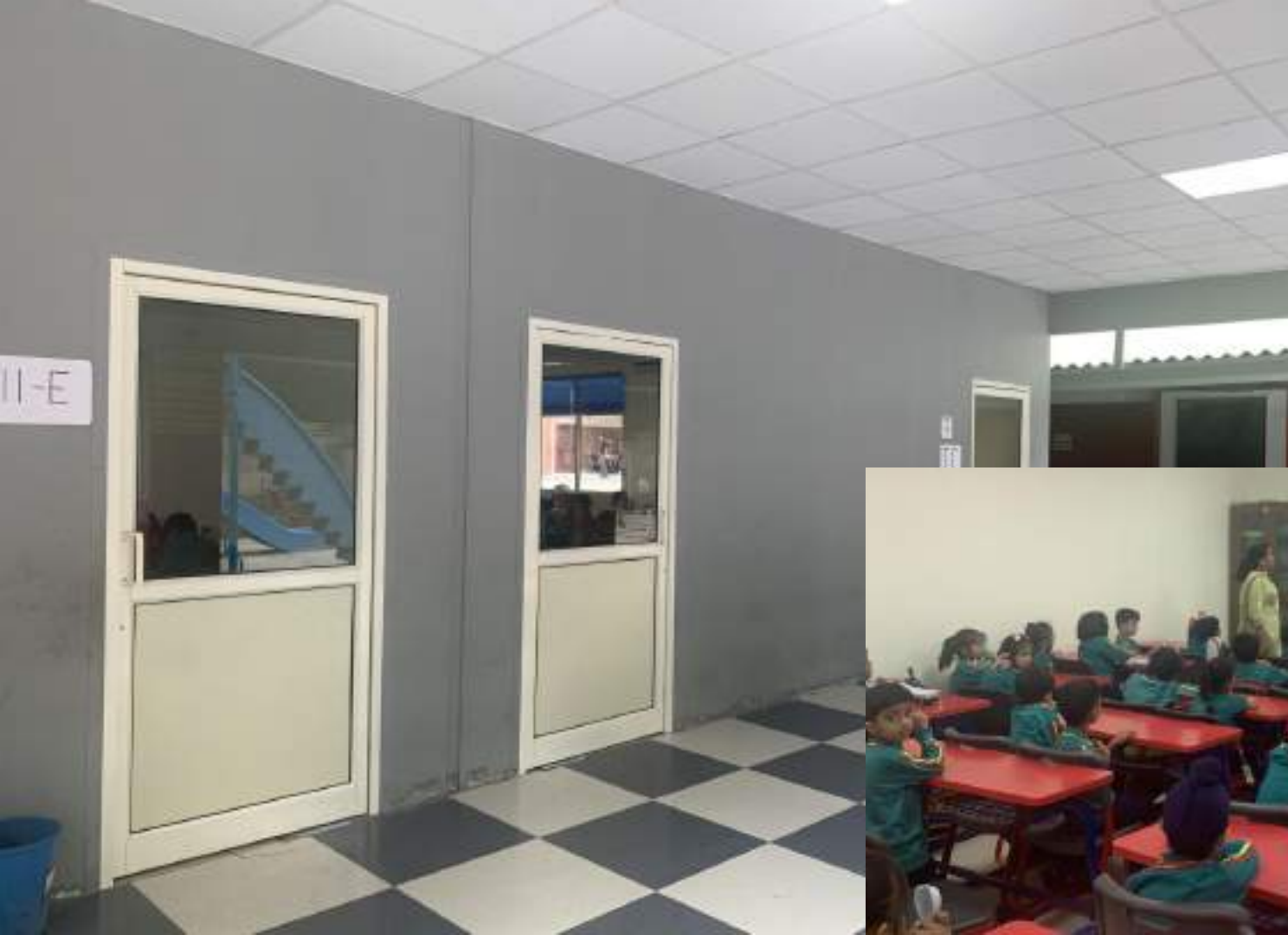
Porta Cabins in Temporary Block at sector 14 Rohini.
