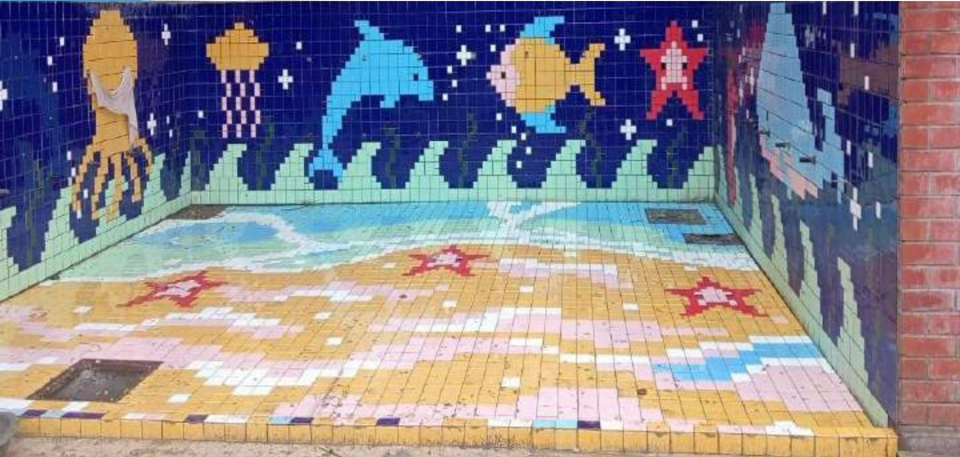
Renovation of Swimming Pool – Outer Shower Area
