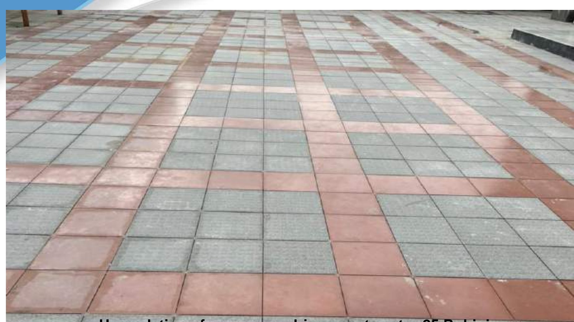
Upgradation of paver near driveway at sector 25 Rohini.
