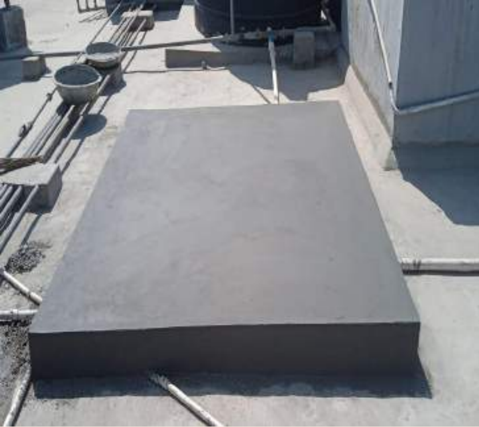
Chillar Plant Foundation Block 1 and 3 roof, Sector-14-work in progress
