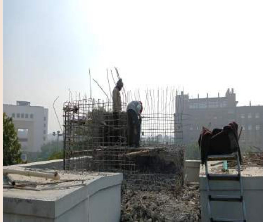
Dismantling of cemented water tanks and fixing of sintex tanks at Block I, Boys' and girls' toilet-work in progress
