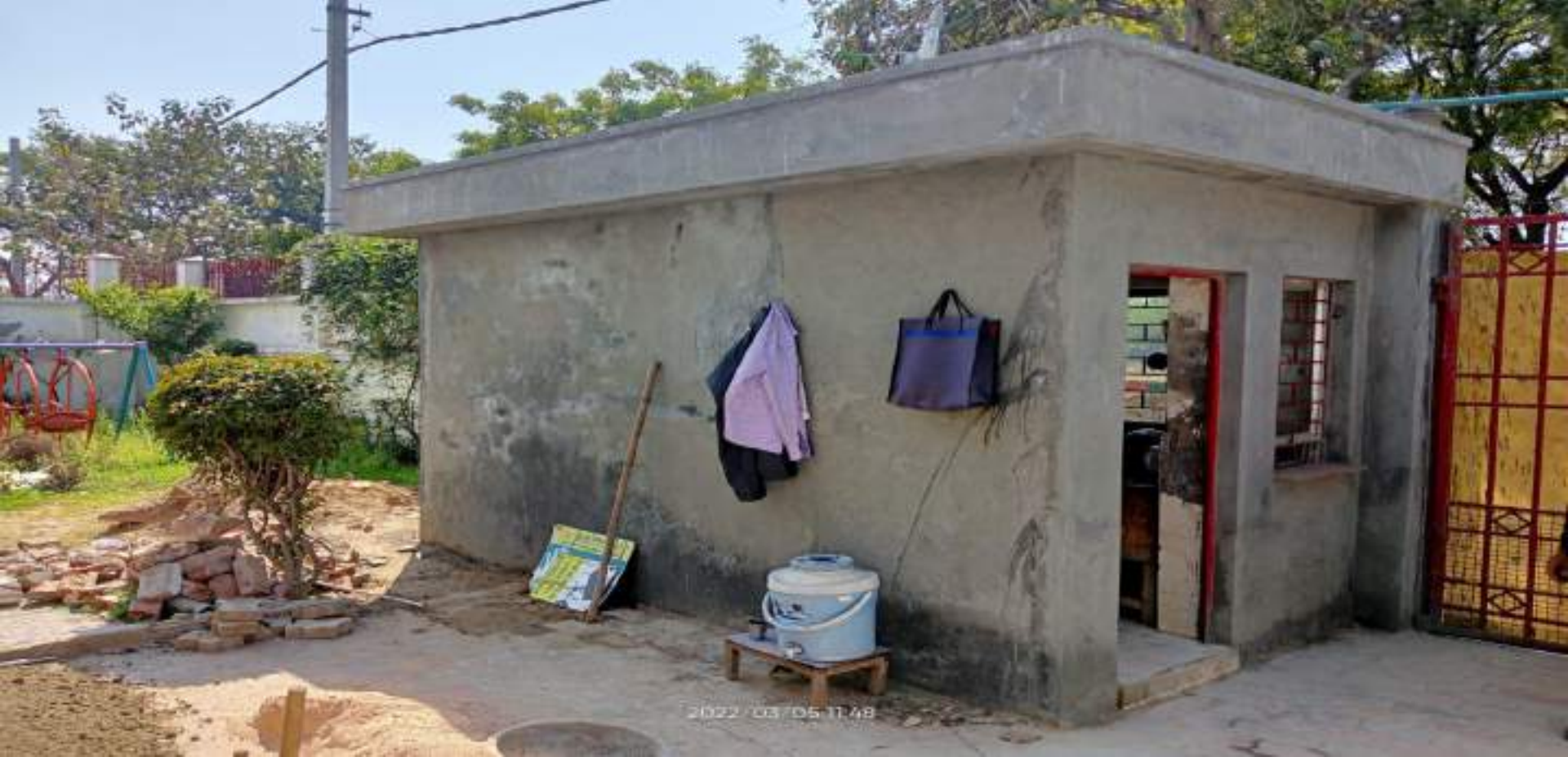
Upgradation of Guard room, Sector 25 -Work in progress
