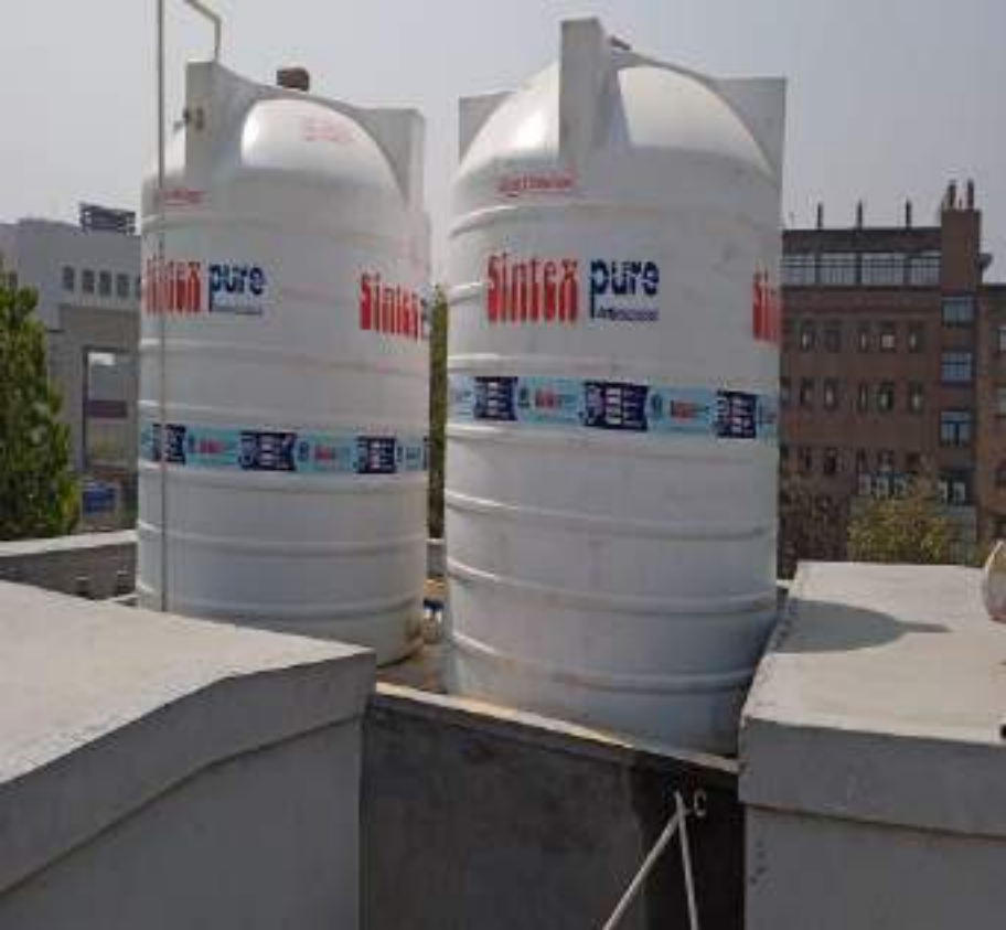
Dismantling of cemented water tanks and fixing of sintex tanks at Block I, Boys' and girls' toilet-work in progress
