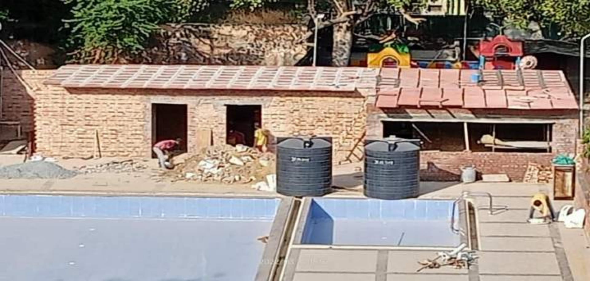
Upgradation of Swimming pool-Work in Progress
