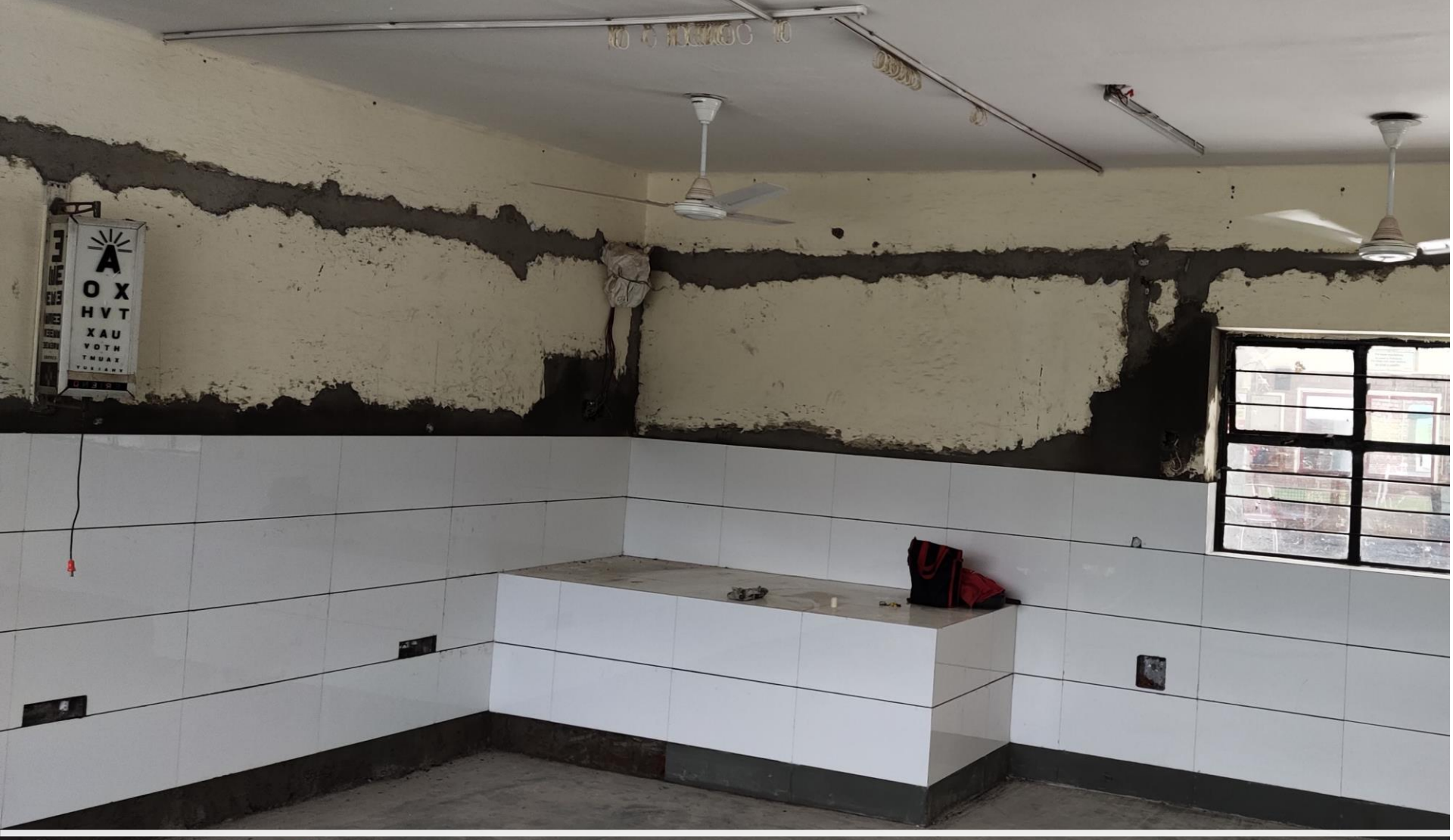
Renovation of Medical Room at Sector -14
